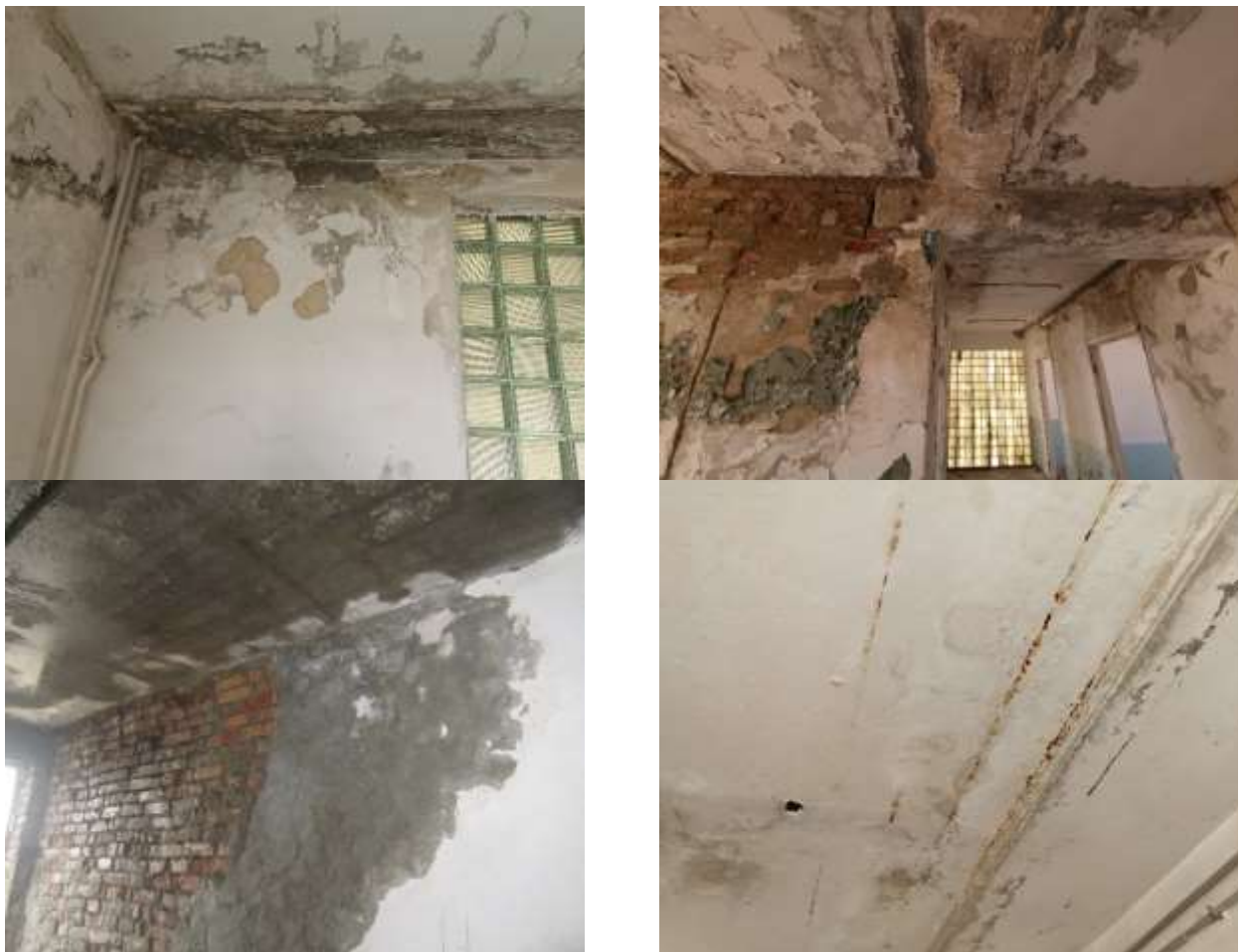
Fig. 1. Damage to the wall and roof slab as a result of the structure getting wet.
